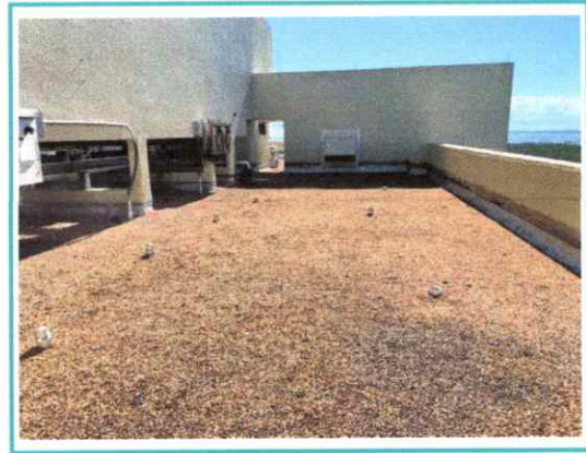
6. Overview of roof system looking S. from W. side center
