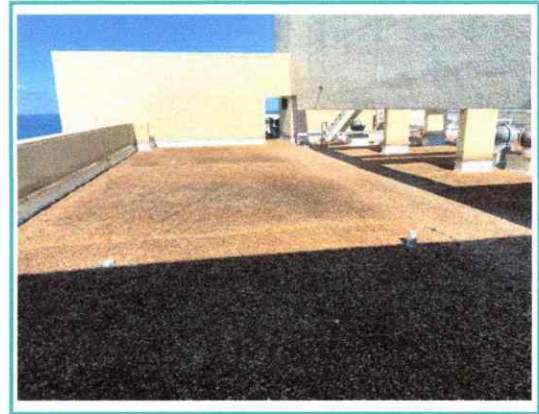
4. Overview of roof system looking N. from W. side center
