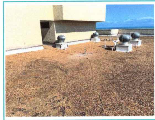
8. Overview of roof system looking NE. from SW. corner
