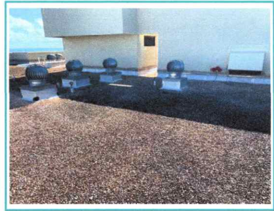
2. Overview of roof system looking SE. from NW. corner
