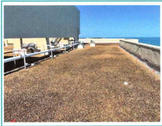
3. Overview of roof system looking N. from E. side center
