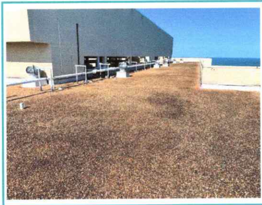
7. Overview of roof system looking N. from SE. corner
