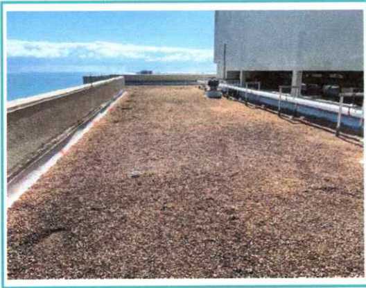
5. Overview of roof system looking S. from E. side center
