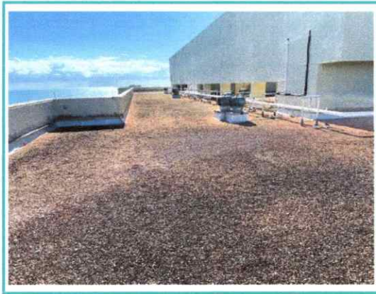
1. Overview of roof system looking S. from NE. corner
